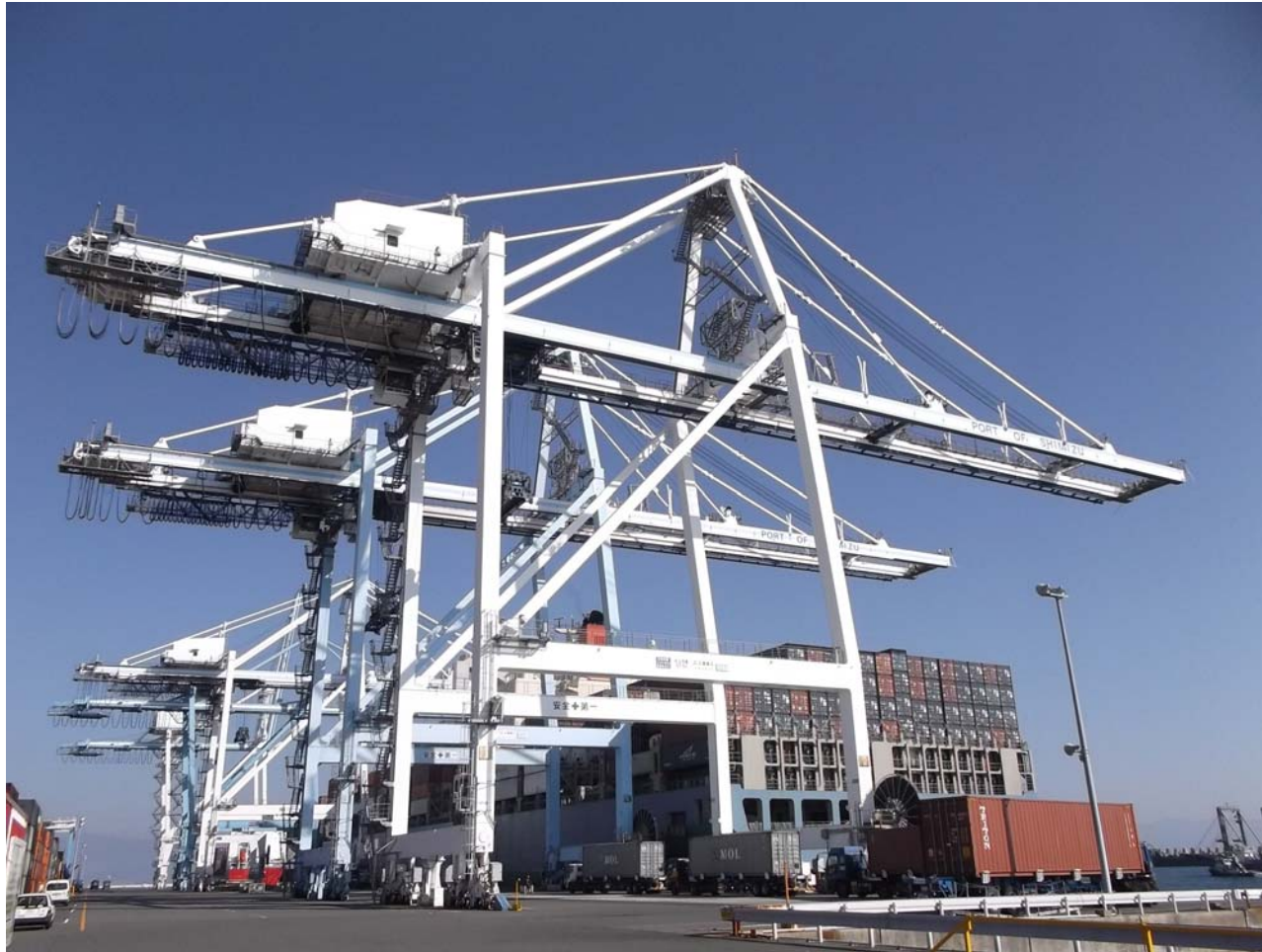
State-of-the-art gantry crane with base isolation system
