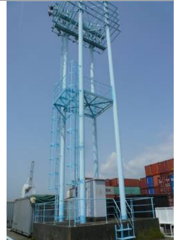
Tsunami evacuation center (floodlights)
